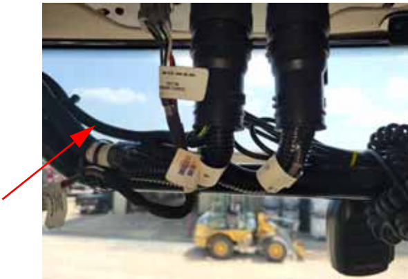
FIGURE 20. Secure Cable with Tie Straps
